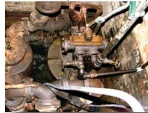
The Shone ejector has no known lifetime. The first units installed in the US over 100 years ago are still in operation. It is designed for extreme dependability in pumping jobs
