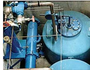
sewage and wastewater using a simple fill/discharge operating cycle using pressurized air or steam. Typically located in the basement of the building, sewage flows by gravity into the cast iron receiver pot.
