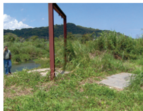
Plant raw water intake caisson
